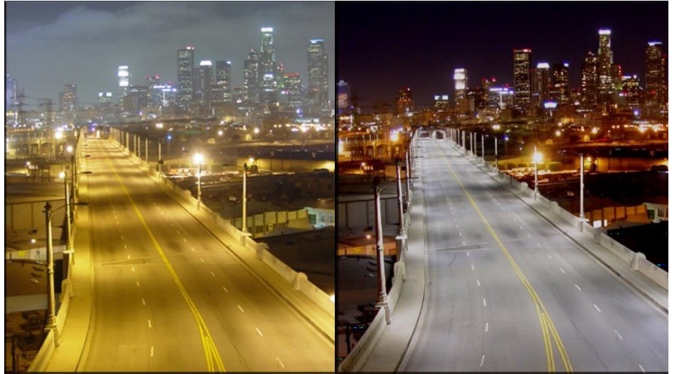
Before and after pictures of replacement lighting at the 6th Street Bridge over the Los Angeles River. The second picture shows improvements in some aspects of light pollution, as light is not directed to the sides and upwards from the upgraded fixtures, reducing skyglow. However, it also shows the use of brighter, whiter LEDs, which is not generally ideal, along with increased light bounce back from the road. Image Credit: The City of Los Angeles
